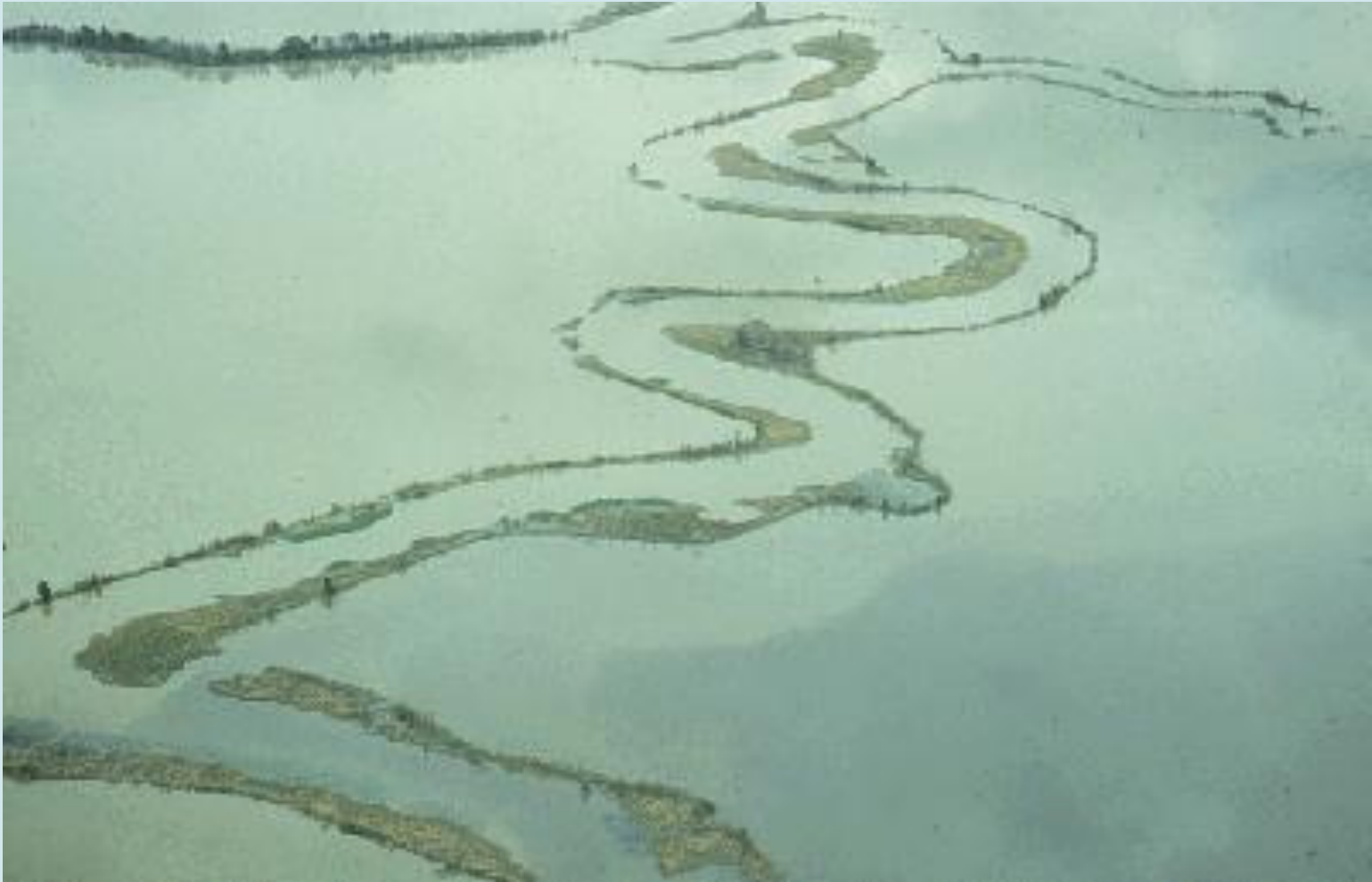
Mississippi river levee banks exposed above floodwaters
