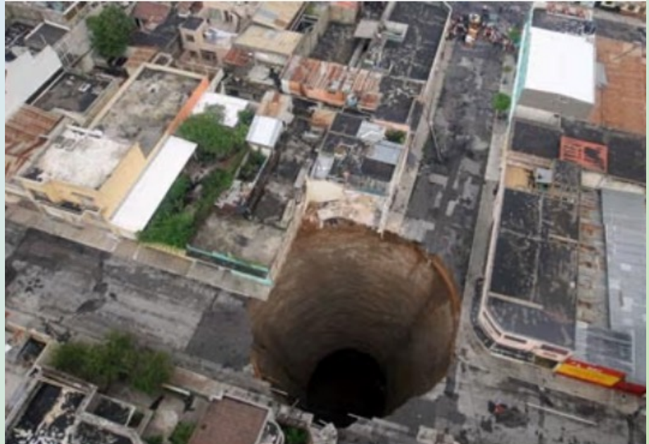
Sinkhole Guatemala City, 2010
